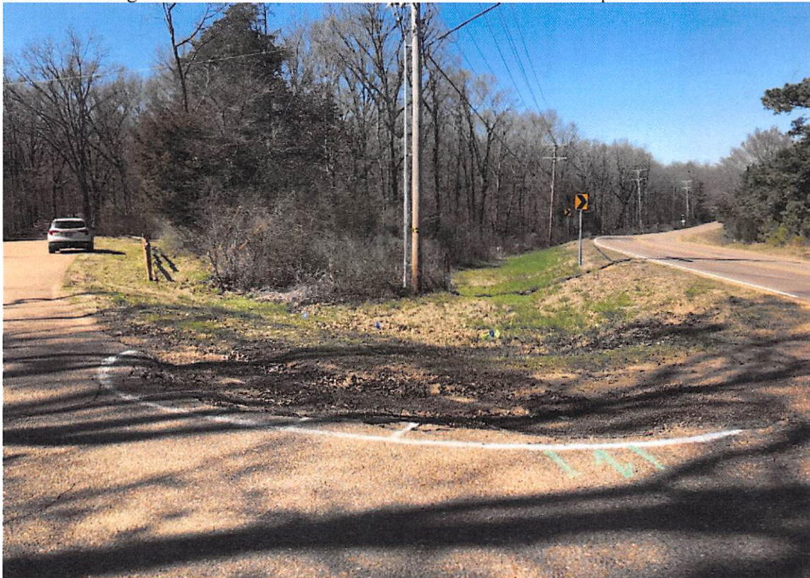
Below: Looking north on Catlett Road from Luebirdia Lane and at broken pavement in radius.
